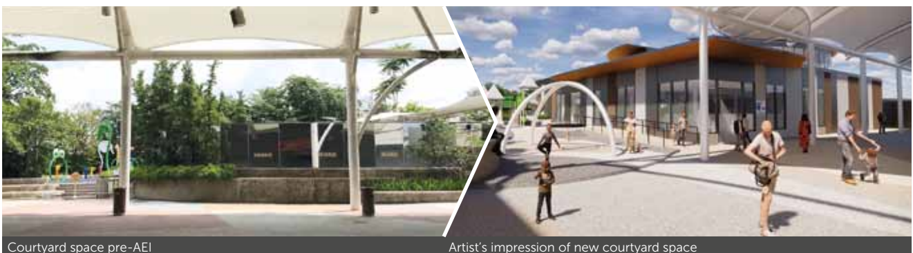
Courtyard space pre-AEI
