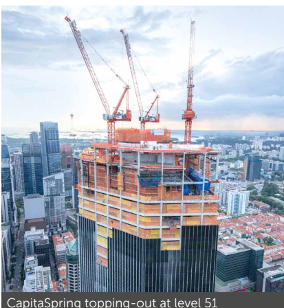
CapitaSpring topping-out at level 51
