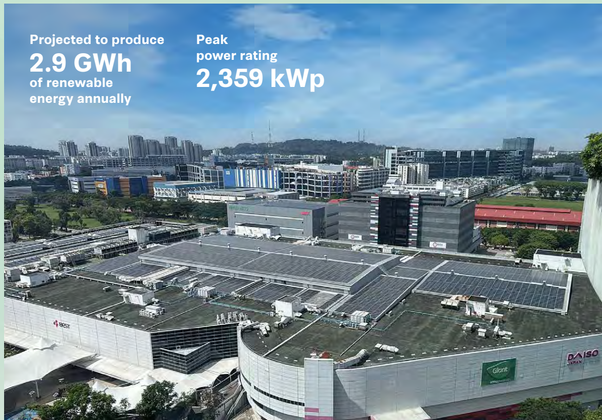
▲ Harnessing renewable energy through solar panels on IMM Building's rooftop.
